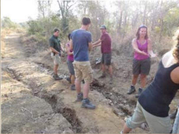
The team carried out some great **Road maintenance** this month, repairing damage caused by the rains back in March. Huge gullies were created which need fixing up before we receive the next rains. The bulk of the hole is filled with small rocks collected from the river. Gravel is collected next and used to fill in all the gaps.
